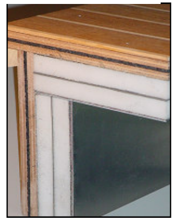
Bulkhead and Cabin Soles
